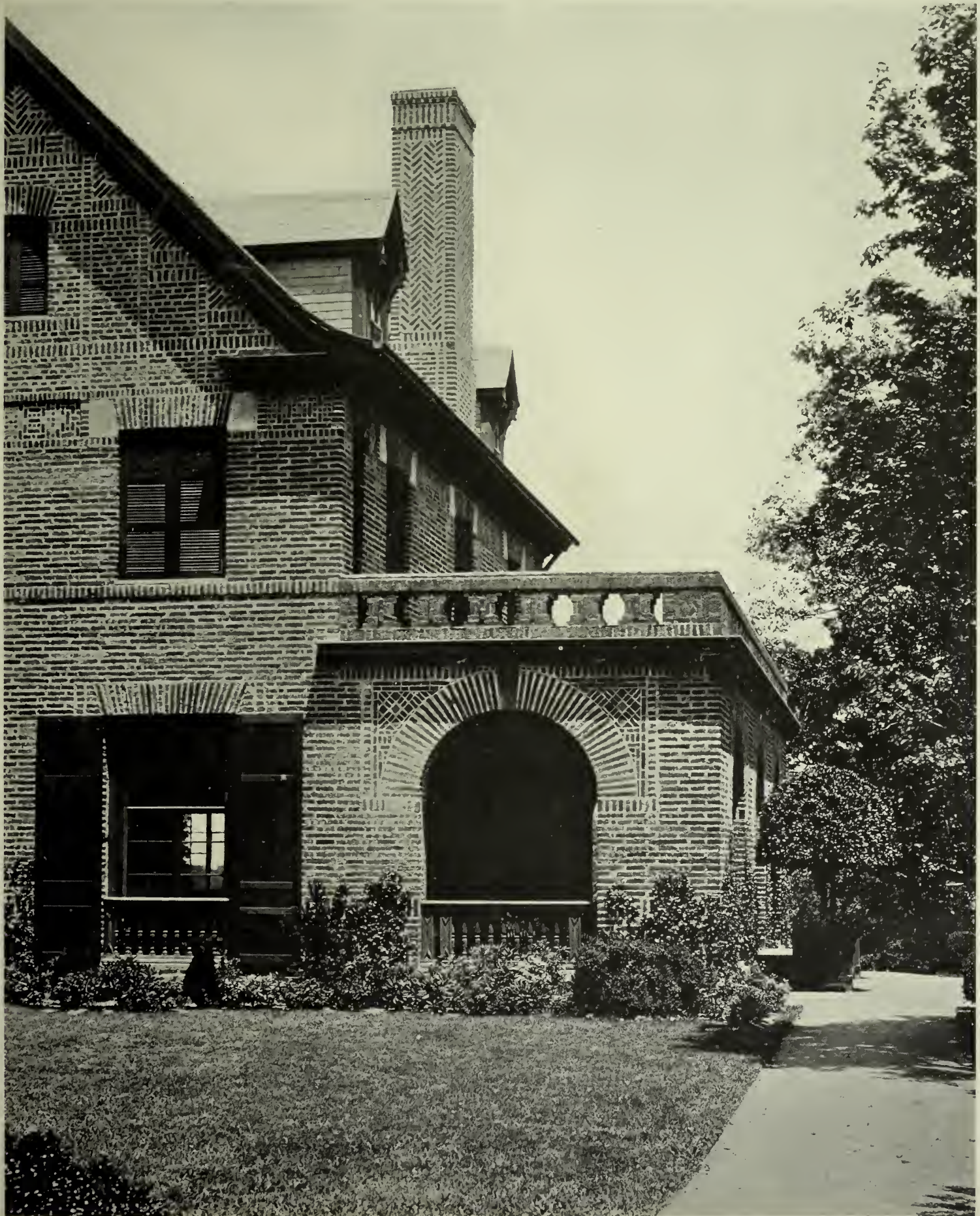
DETAIL OF LOGGIA OVERLOOKING GARDEN.
